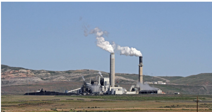
Figure 10 Terrapower's SFR will drop in replace coal heat for this steam cycle electricity plant in Kemmerer, WY.
