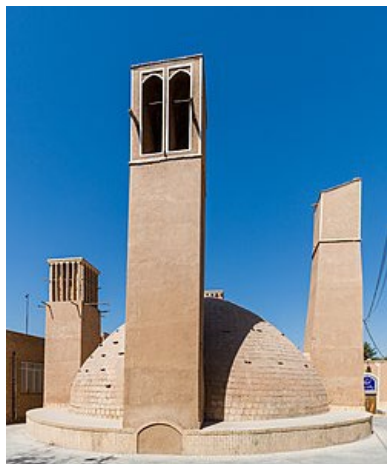
Figure 3 Left: Ancient cooling towers that capture wind in Yemen. Right: Sodium Fast Reactors use natural convection of liquid sodium in the reactor vessel ‘bath’ and ambient air surrounding the vessel and flowing freely to tower inlets and outlets, in order to cool down an overheating incident.
